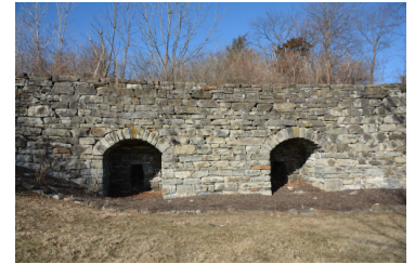
The Muscnetcong River Valley Double Lime Kiln on Rt. 31 may have served several farms.
